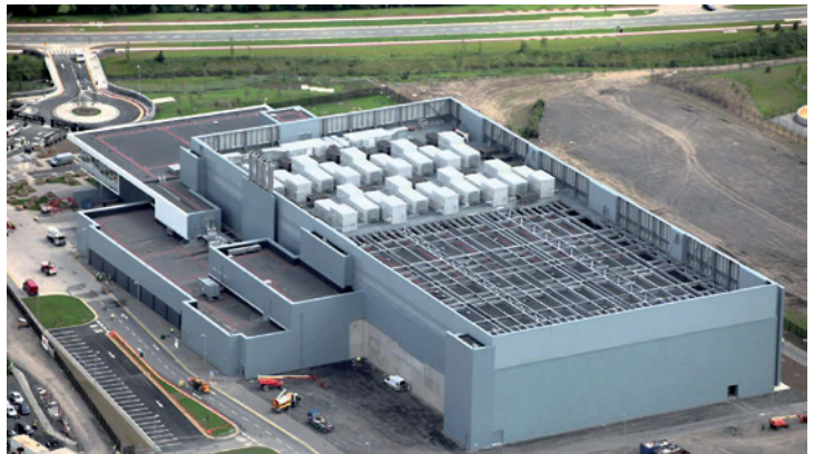
Abbildung 1: Das Azure-Datacenter in Dublin, Irland ( global-foundationservices.com )
